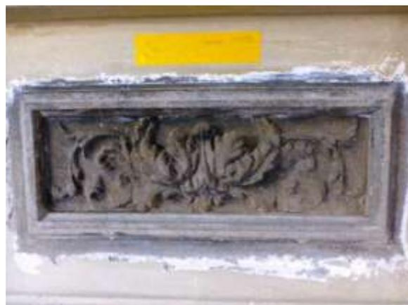
Now the paint has been removed work has started on repairing damaged render, removing rusting iron, stitching structural cracking and rebuilding missing and damaged decorative elements. Carefully colour matched hydraulic lime render is being used for these repairs.
