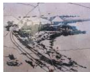
Two of the damaged tiles
