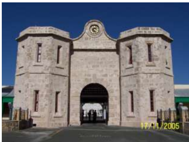
The recently conserved Fremantle Prison Gatehouse with its original clock. (Photo courtesy Fremantle Prison).
